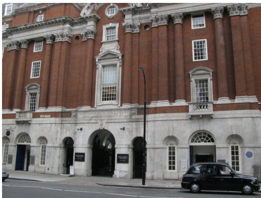
The British Medical Journal was a Funnelback client. We went to project meetings in this impressive building. There is another plaque further along the wall, in memory of the 13 people who died when a bus was blown up outside this building in 2005. Medical staff in the BMA building rushed out to render assistance.
