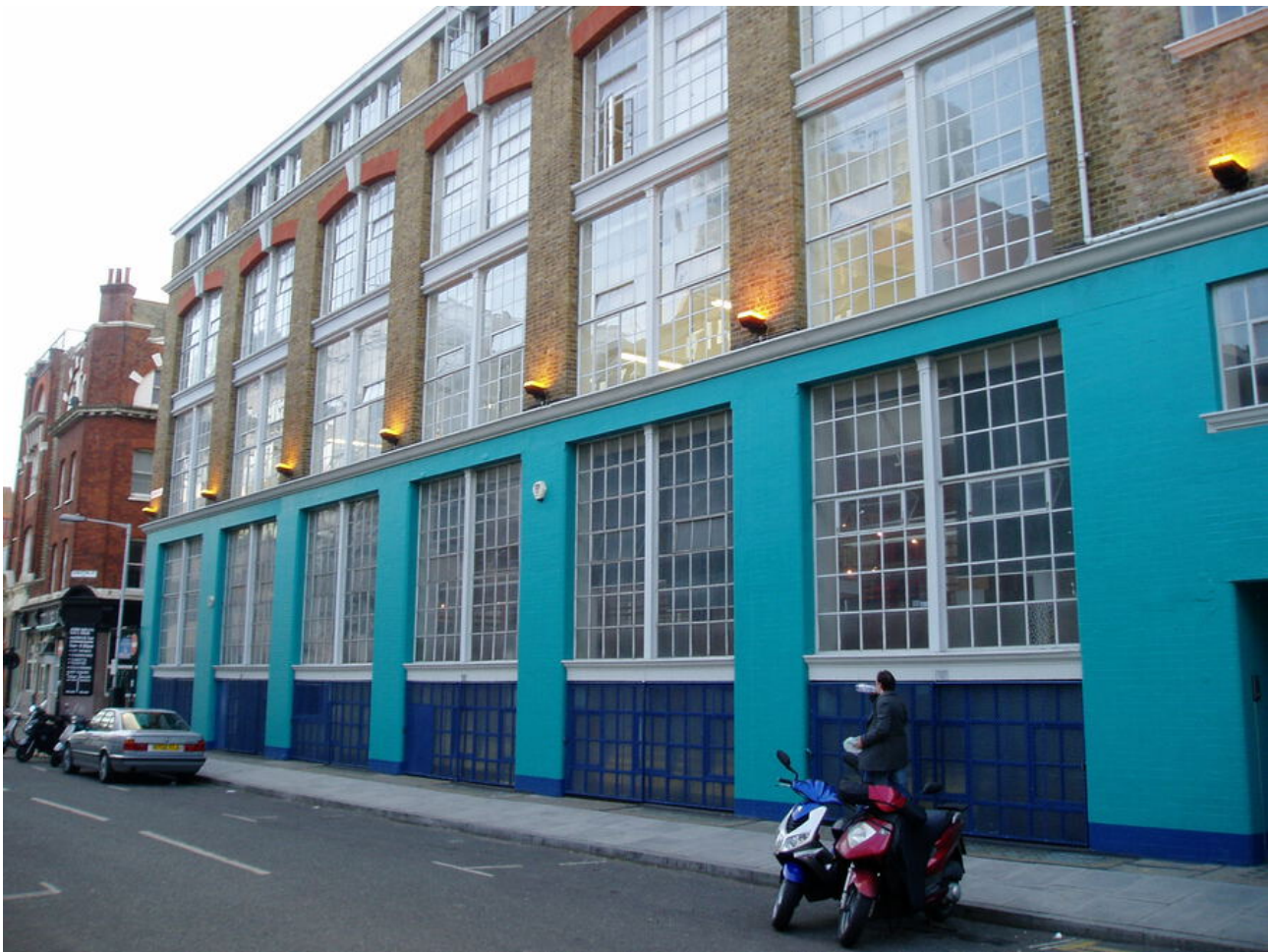
2009: Zetland House in Clifton St, Shoreditch EC2A 4HJ. The building originally housed a note printing works for the Bank of England. The original Squiz UK office was on the very top floor. Steve Morgan eventually leased one of the parking spots seen here in order to park his BMW Z4 sports car.
