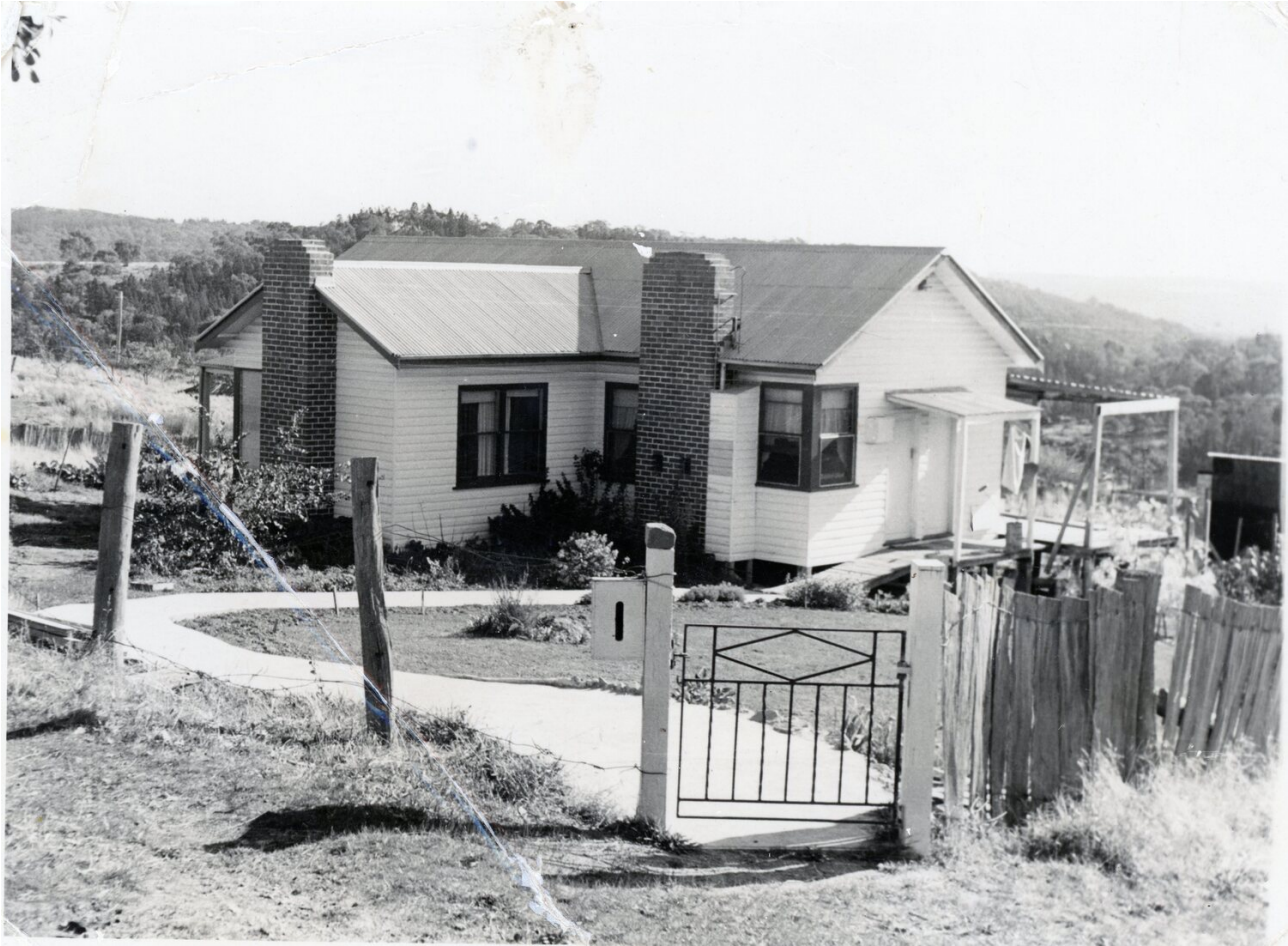
c. 1956: The house at 49 Camp St – Lived in but lots of work to be done. The little porch was in the process of being replaced by a verandah and the house was in process of acquiring a magnificent garden. At some stage the height of the kitchen chimney was increased at Uncle Skipper's suggestion to solve Margaret's complaint that it wasn't burning properly.
