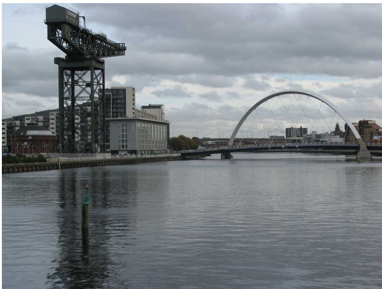
2011: The Finnieston Crane, 45 capable of lifting 175 tons and used for loading locomotives onto ships; the Mint hotel where I stayed; and the Squinty Bridge, aka the Clyde Arc. 46
