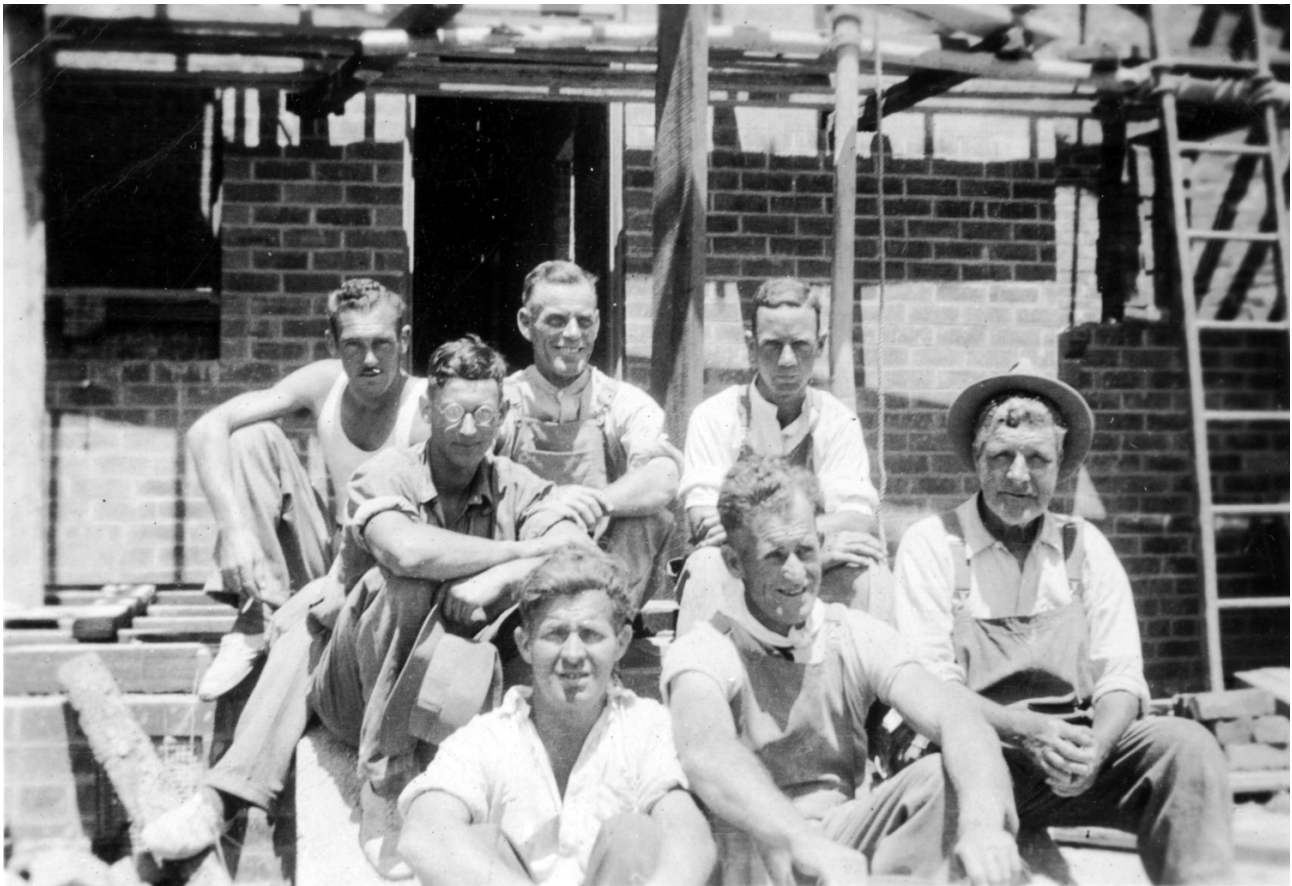
Building the State Savings Bank residence at Beechworth. Ern middle left, Skipper back right.
