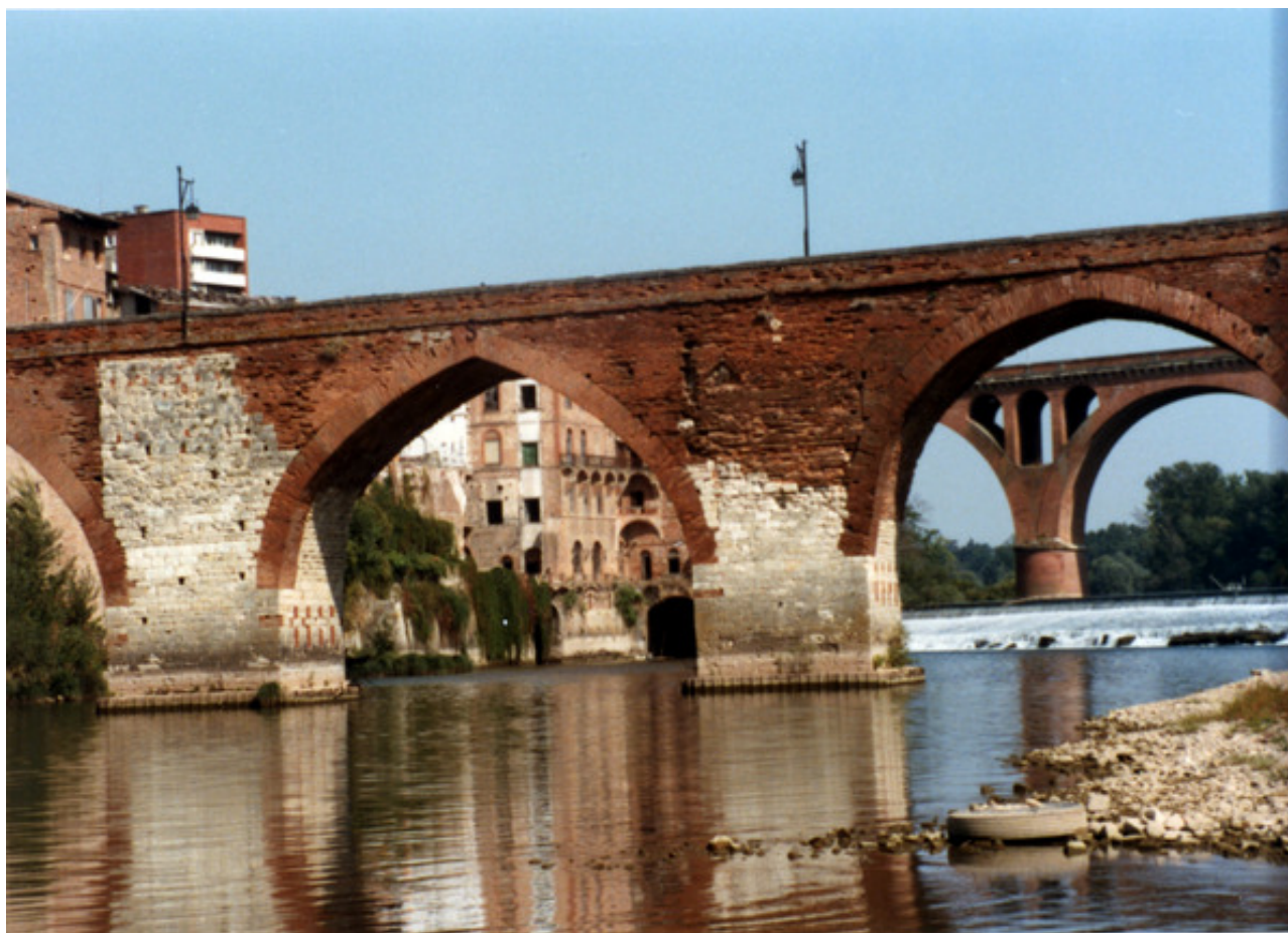
1985: Bridges in Albi, France. Note the use of brick and the two styles of arch.
