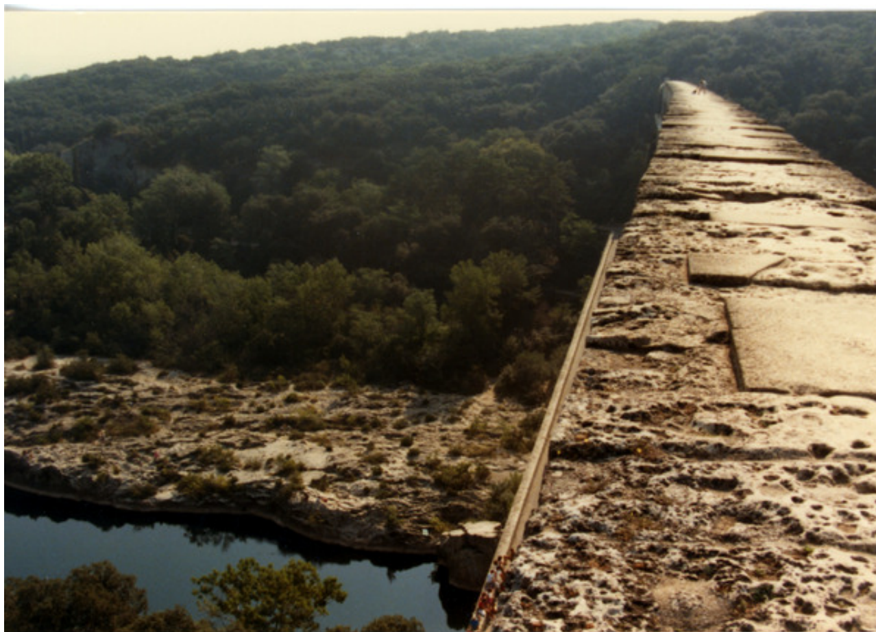
1985: The flagstones covering the water channel on top of the Pont du Gard. Nîmes, France.
