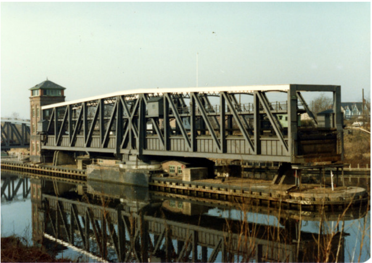
1979: The canal overpass, rotated so that boats on the main canal can pass on either side. Manchester, England.
